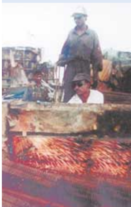
Gas cutting operation
