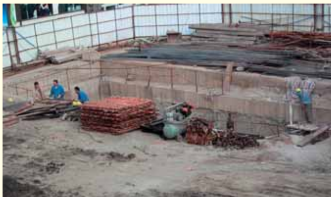
Construction site in Jiangsu Province, P.R. China. (Photo by Seppo Olkkonen)
